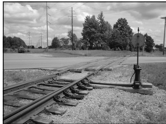
A&L Rail Project On Track
